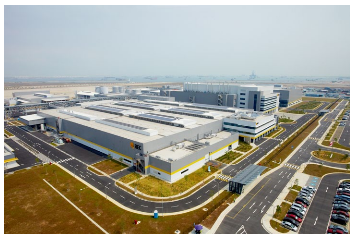
The complete system installed at REC's integrated manufacturing facility in Tuas, Singapore.
