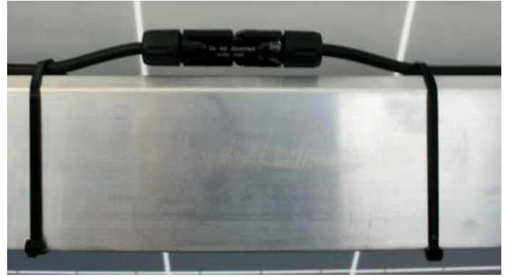
Fig. 10: Best practice installation of a connector allows air circulation around the connector body with connector secured either side
