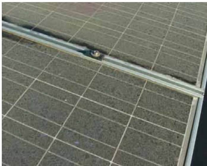
Fig. 1 An example of dust build-up on solar panels over time.
